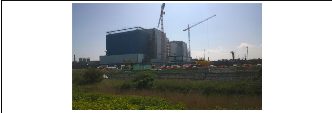
Figure 33 – Decommissioning Bradwell A Power Station in the UK [25].
