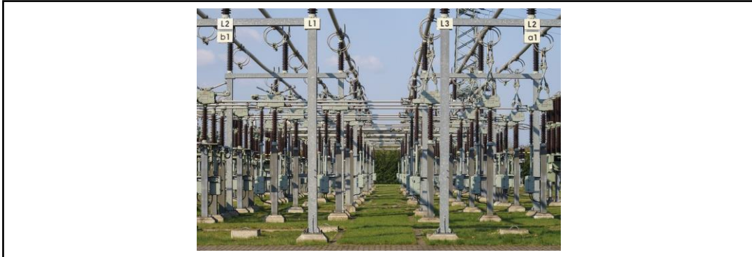
Figure 18 – Example of industrial transformers [11].
