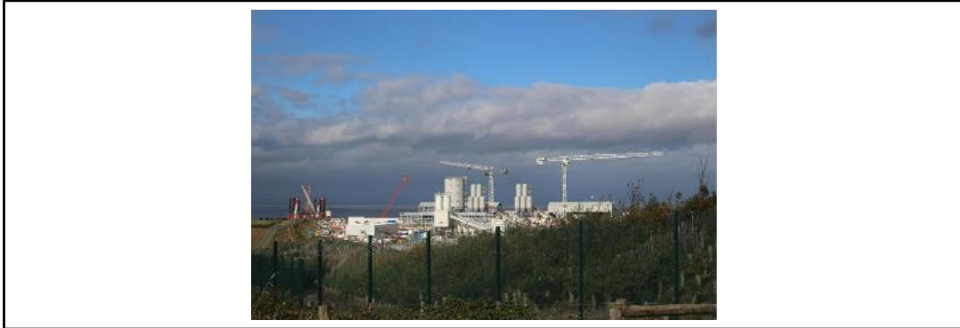
Figure 31 – Early stages of construction of Hinkley Point C power station [23].
