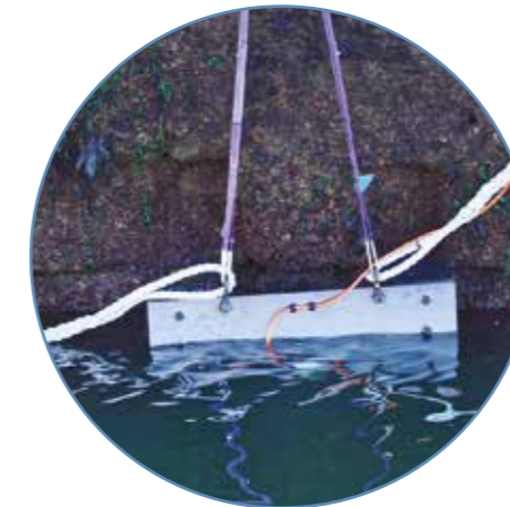
Test piece being lowered into position
